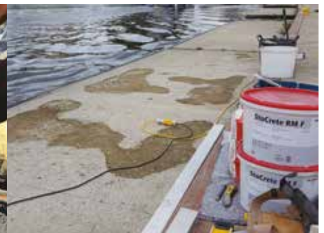
Quick and easy repairs with StoCrete RM F
